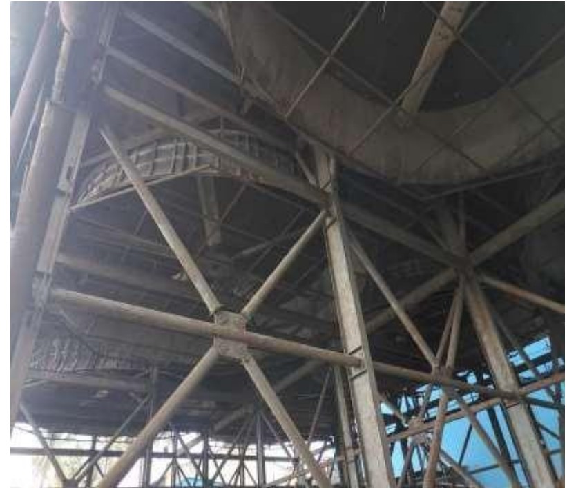
Air Cooled Condenser for 23MW power generation through Bagasse Fired 120 TPH, 125 ata Boiler.
