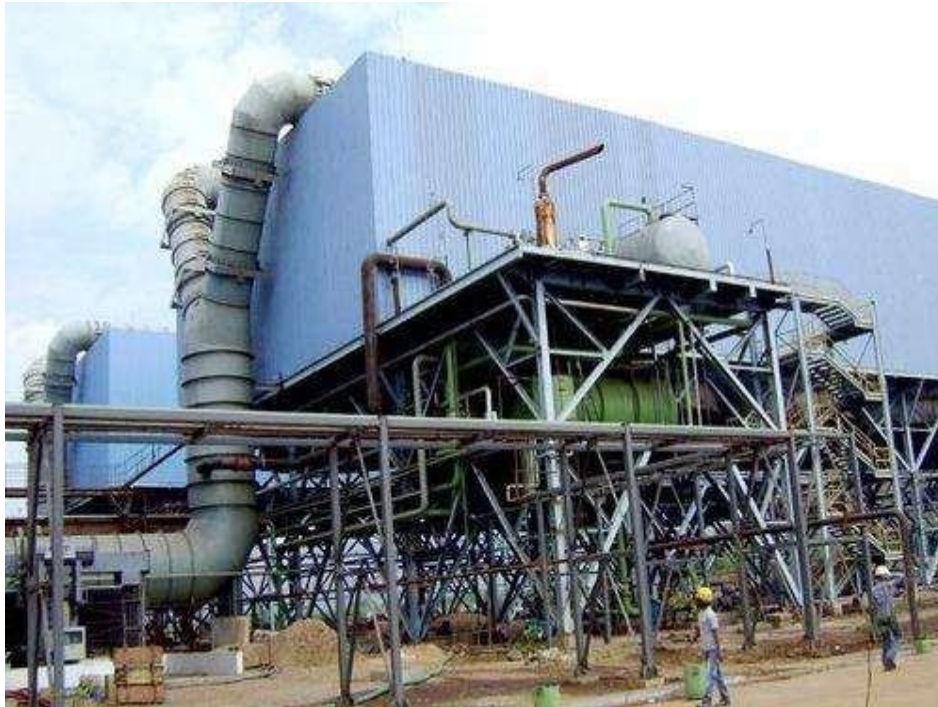
Air Cooled Condenser for 23MW power generation through Bagasse Fired 120 TPH, 125 ata Boiler.
